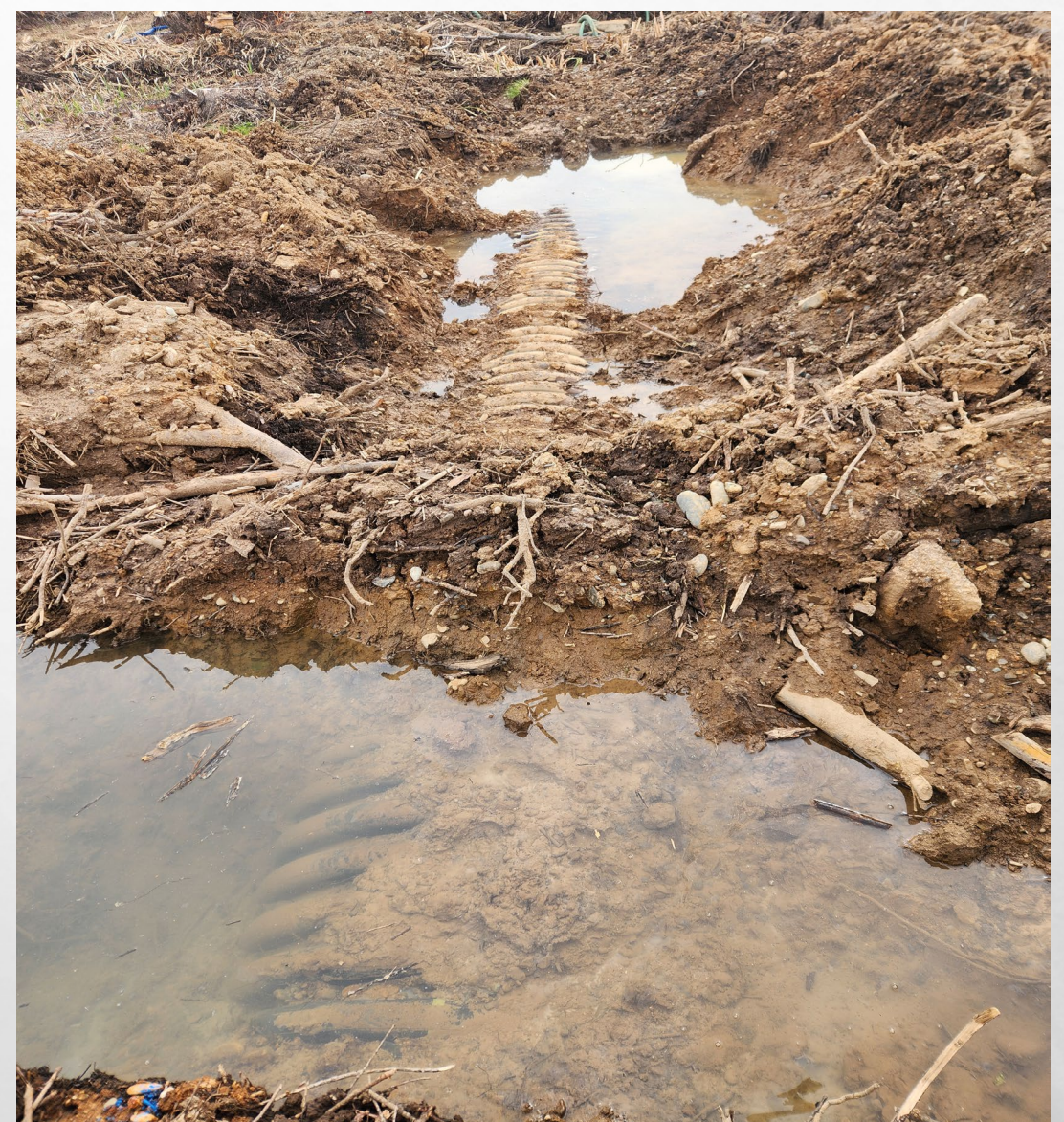
Disconnected Joint
