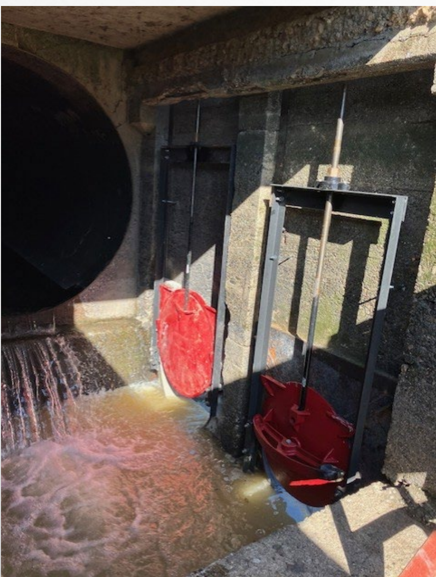
Refurbished Spring Gulch Spill Gates
