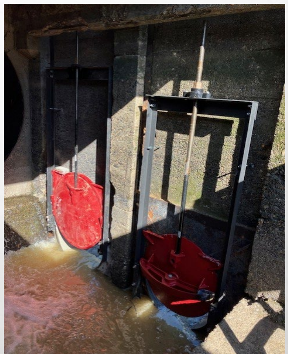
Refurbished Spring Gulch Spill Gates
