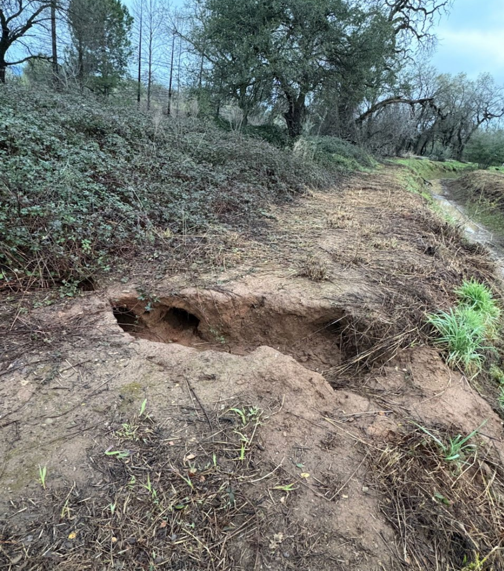
Churn Creek Bottom Main Canal – Rodent Washout
