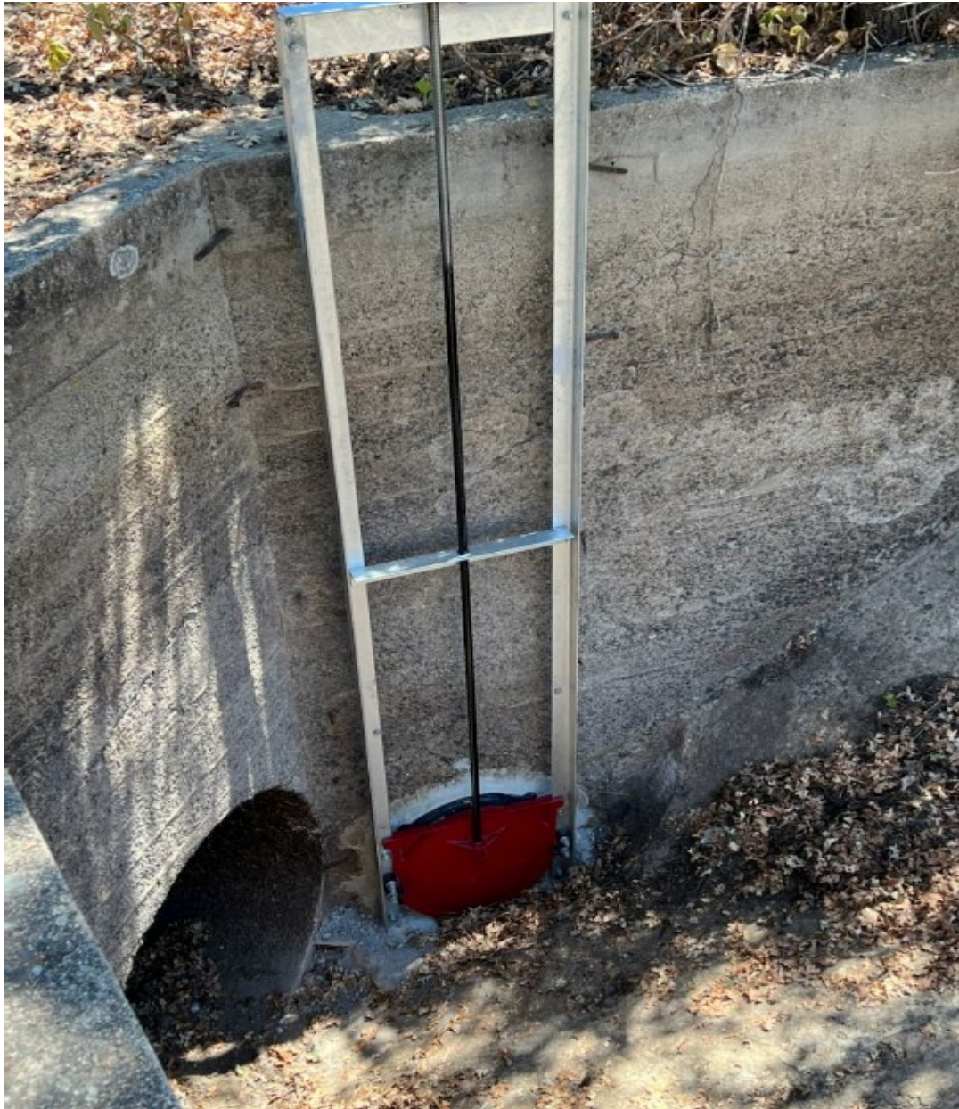
Spillway at Cottonwood Creek
