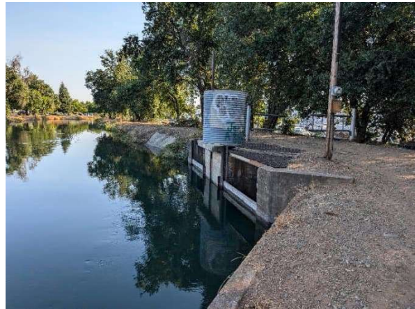
Figure 2-5. Photograph of Existing Canal Spill Looking Upstream
