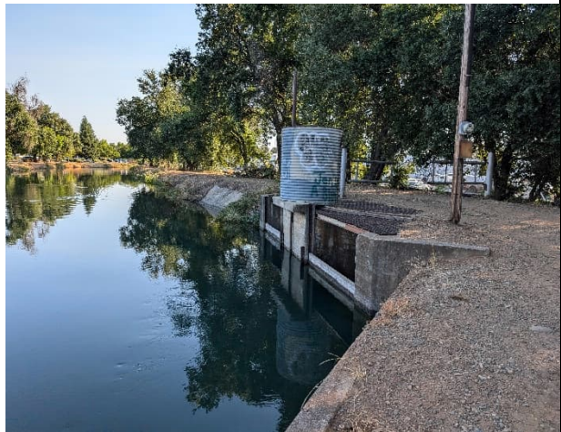
Figure 2-5. Photograph of Existing Canal Spill Looking Upstream
