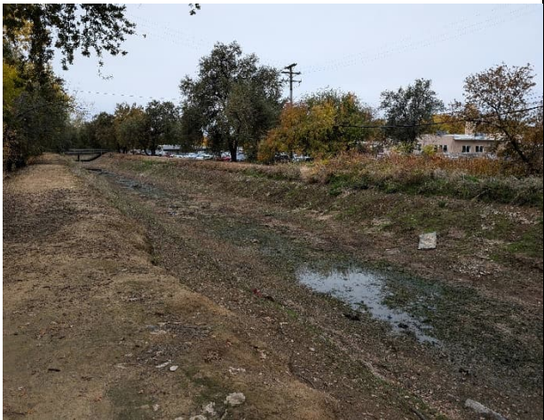
Figure 3-4. Photograph of Main Canal Looking Downstream
