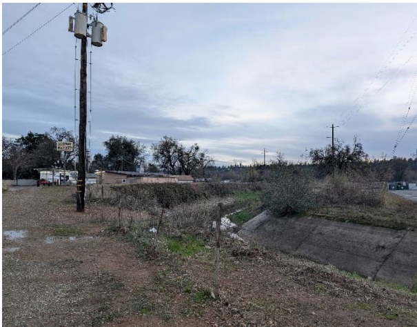
Figure 4-4. Photograph of Main Canal Looking Downstream
