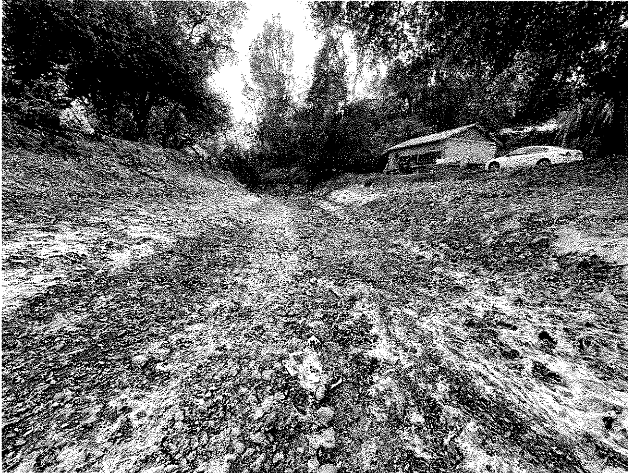
Image 2: Preconstruction condition of canal with relatively shallow right side channel slope
