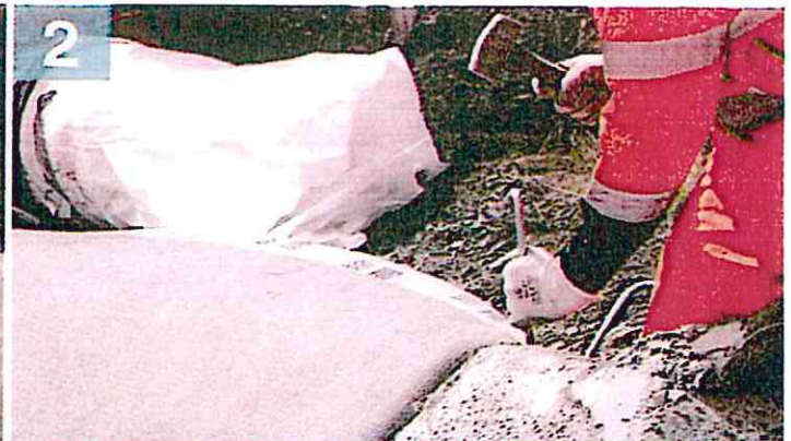
Pegging CCX™ within anchor trenches
