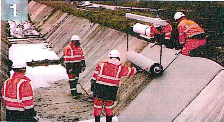
Deploying Bulk Roll of CCX™
