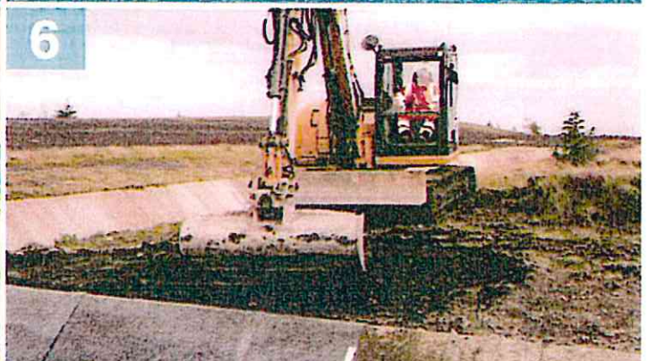
Backfilling anchor trenches to prevent ingress
