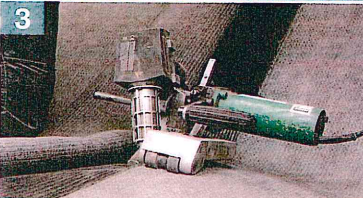
Thermal welding of CCX-B™ LLDPE backing
