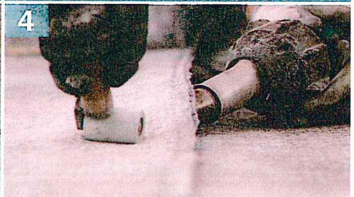
Thermally bonding overlapping layers of CCX™
