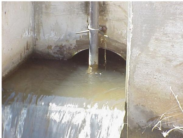
**Figure 7. Weir boards are installed downstream of an open propeller meter. Obviously, these are not high enough to create a full pipe condition.**
