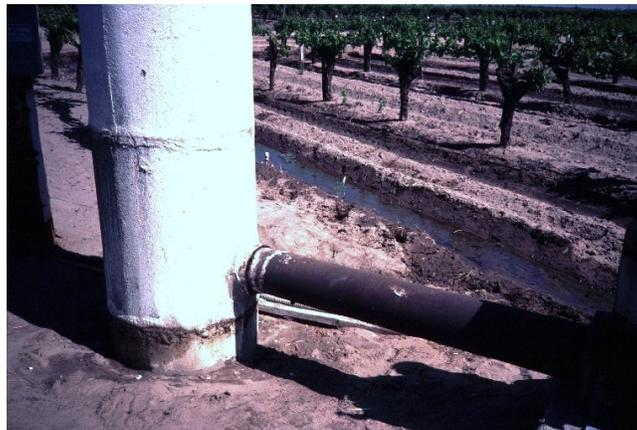
**Figure 47. The discharge pressure of the pump will change over time with this type of direct connection to a standpipe**
