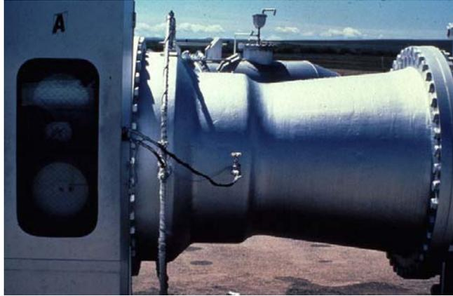
**Figure 11. Large, old venturi and instrumentation at Berrenda Mesa WD pumping plant**
