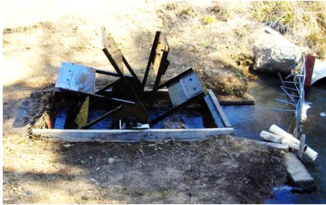
Figure 10. Locally fabricated trash screen in Browns Valley ID
