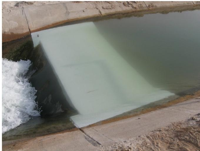
**Figure 40. A flume with an ePaint™ coating to minimize algae growth**
