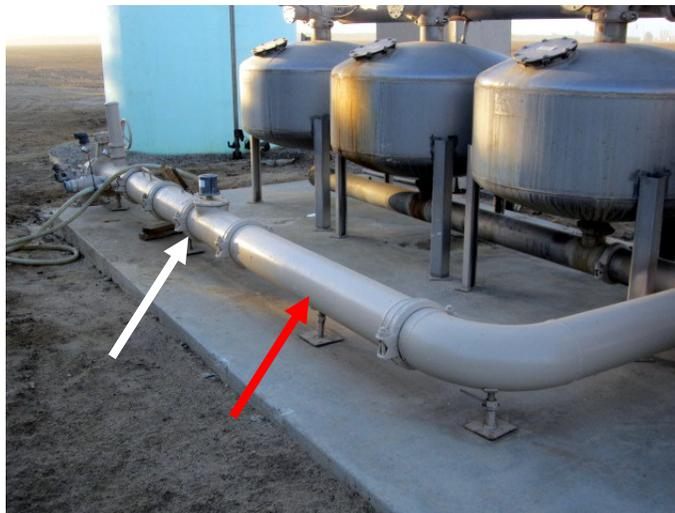
**Figure 3. A propeller meter (white arrow) installed downstream of drip system filters, with a long, straight pipe section upstream of the meter (red arrow)**
