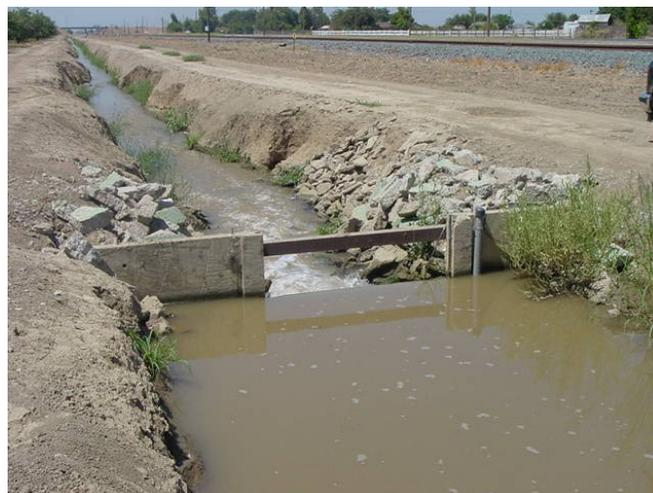
**Figure 44. Example of a rectangular contracted weir**
