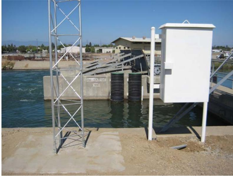
**Figure 3. Automated radial gates on Glenn Colusa ID main canal at IID. Radio tower and instrumental enclosure for a PLC are in the forefront.**
