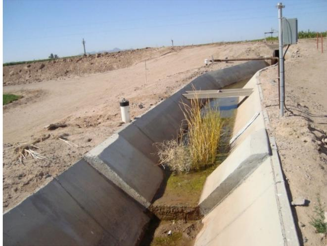
**Figure 39. Flume with expensive monitoring and a slight maintenance problem**
