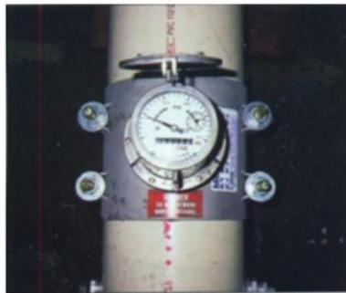
turbulence caused by the valve had little effect on the flow-meter readings.
