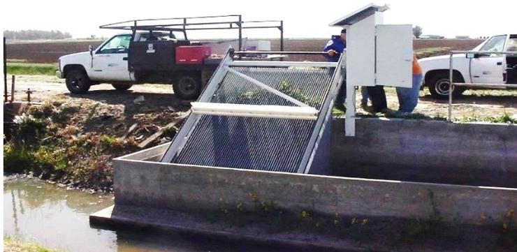
Figure 11. Automatic screen upstream of a turnout in Merced ID. Note the wall that helps prevent sand from entering the turnout.
