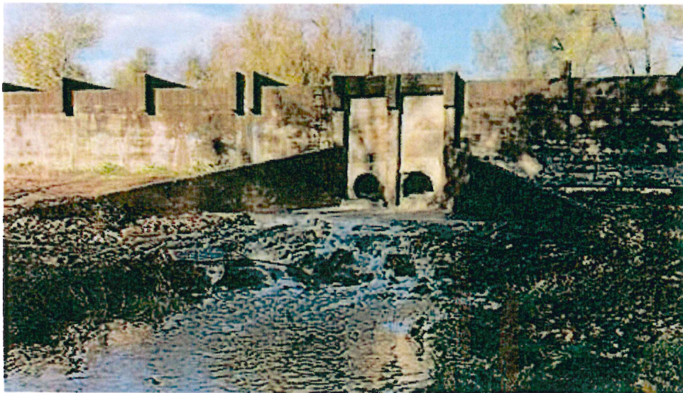
Main Canal at Spring Gulch Vegetation Removal and Spillway Repair
