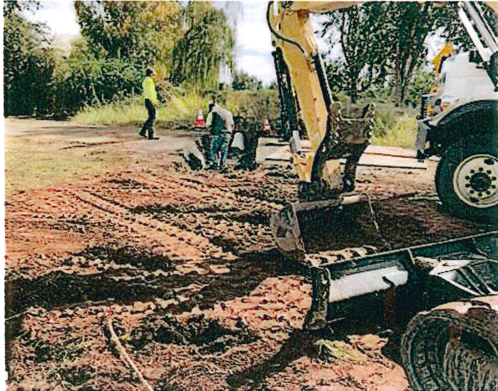
County Staff installing pipe on Venzke Road
