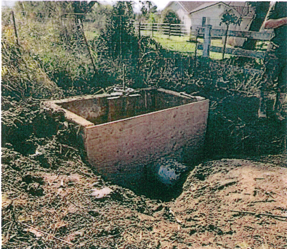
Modifying Distribution Box at Venzke Road
