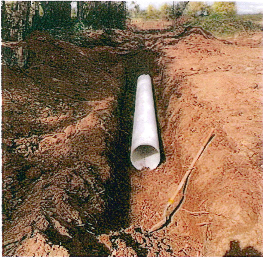
ACID replacing failed concrete pipe and open ditch
