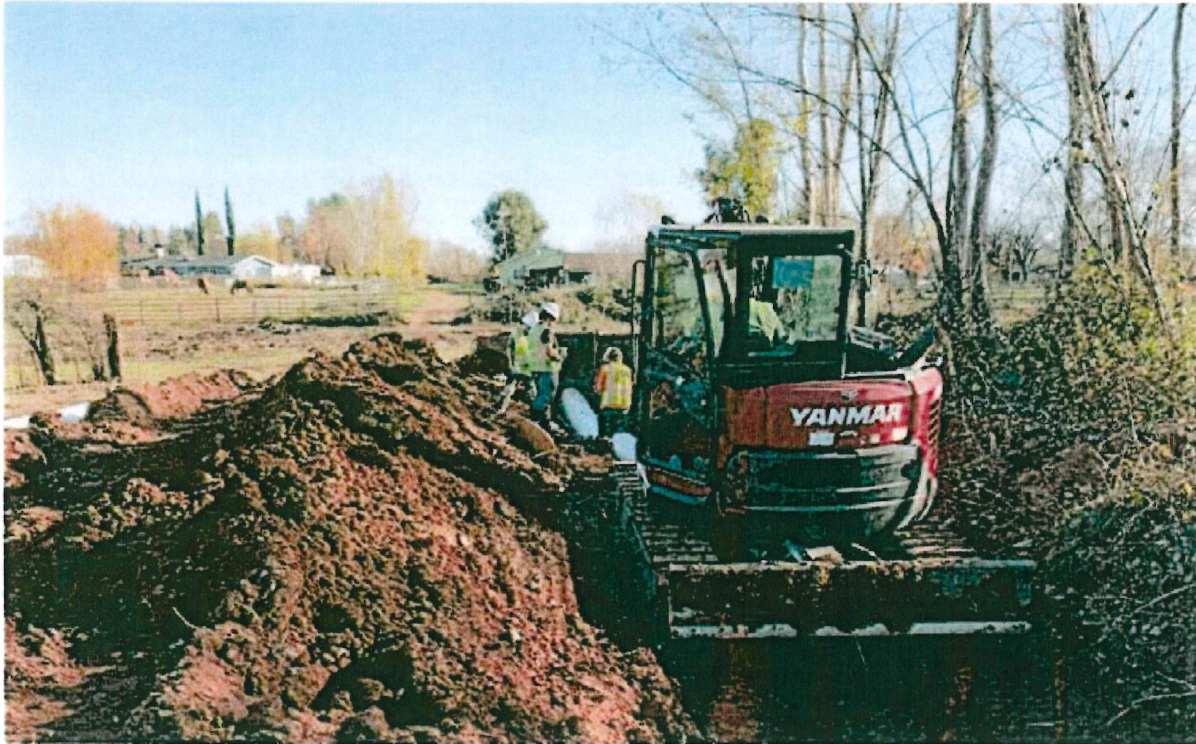
Pipe Installation ACID crew and rented mini excavator on Lateral 33 near Venzke Road
