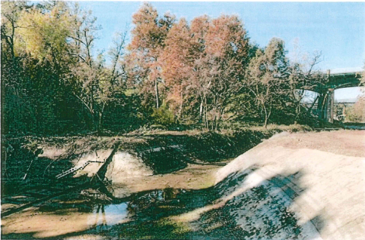
Vegetation Removal at the Dam
