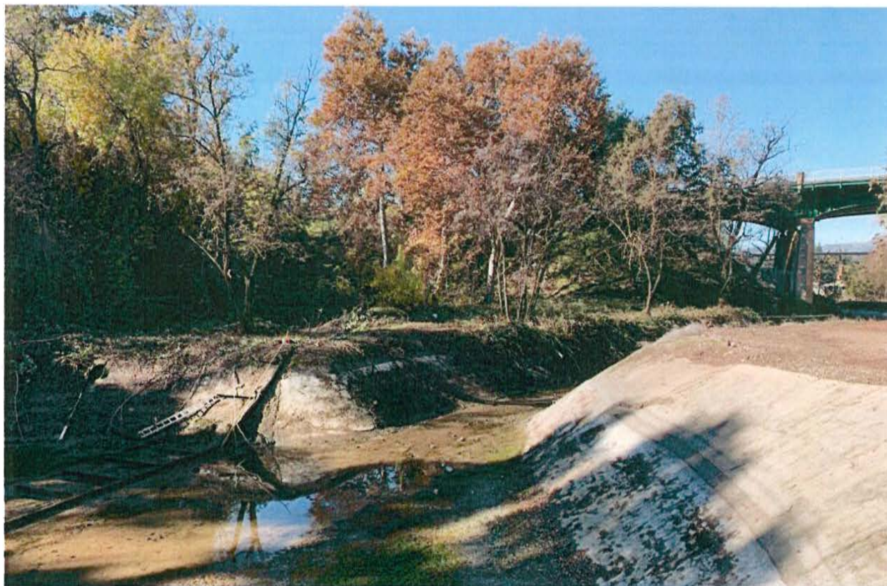
Vegetation Removal at the Dam
