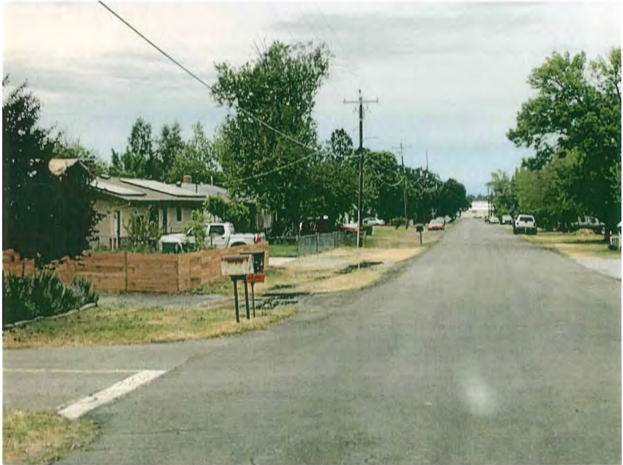
Seepage In the Verdi Vale Area on Hill Street April 24, 2021
