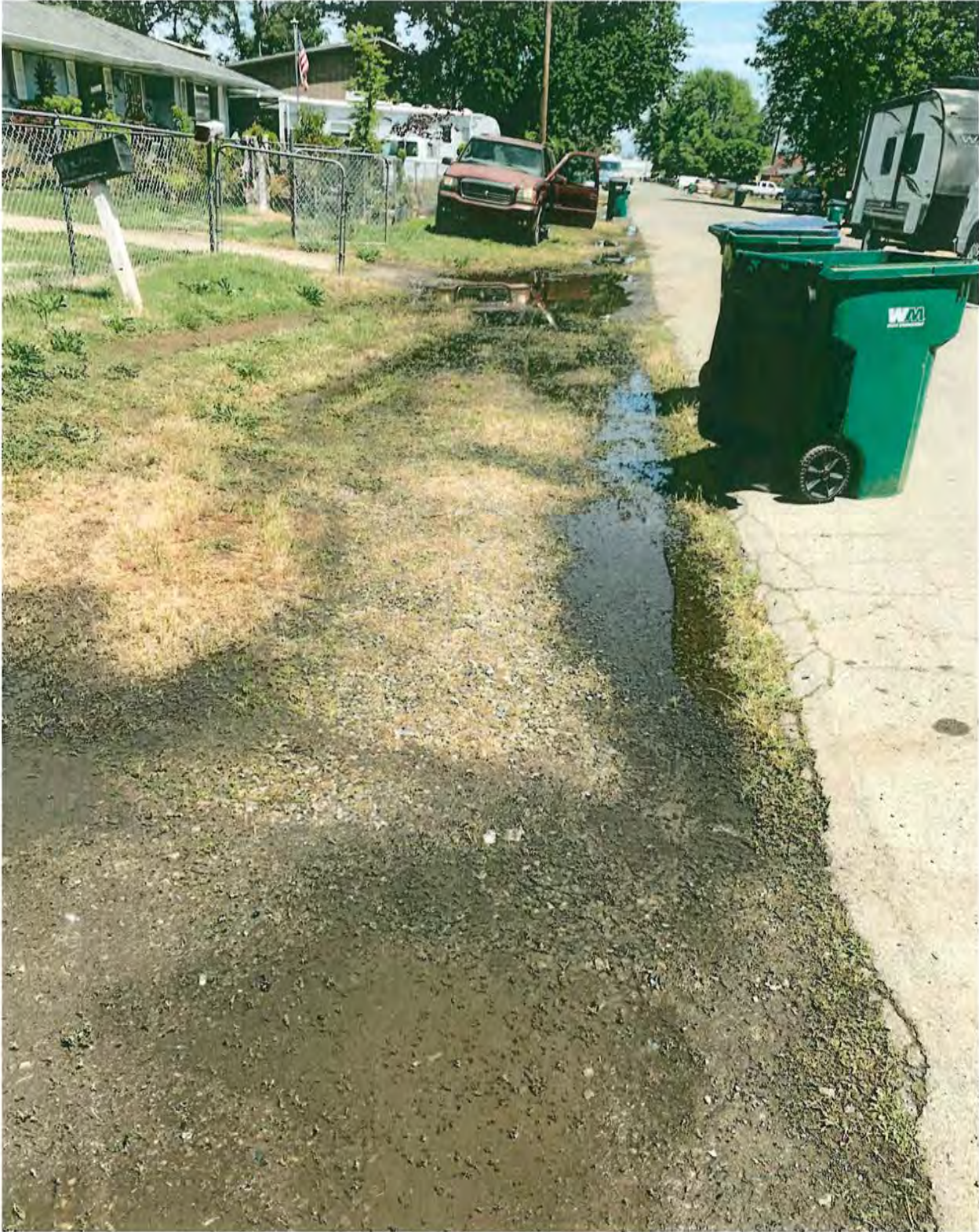
Seepage along Lucille Street on April 29, 2021
