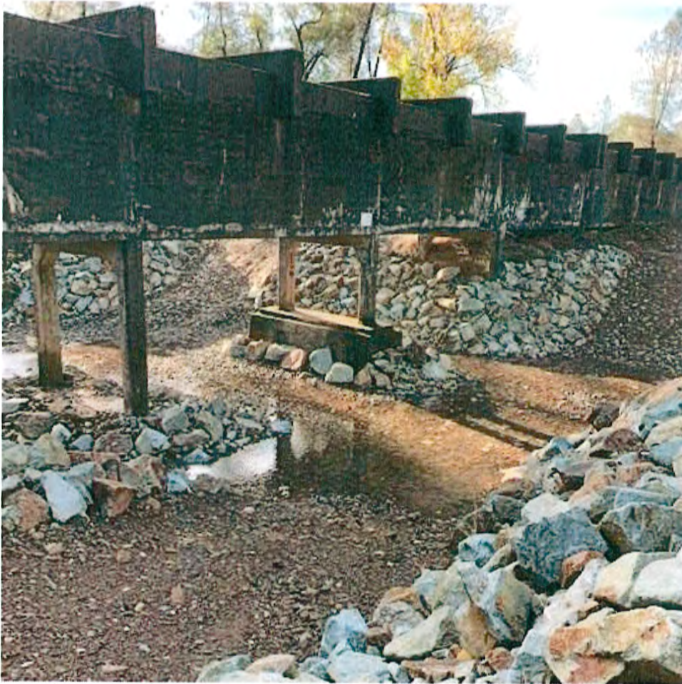
Main Canal at Spring Gulch Vegetation Removal and Foundation Repair
