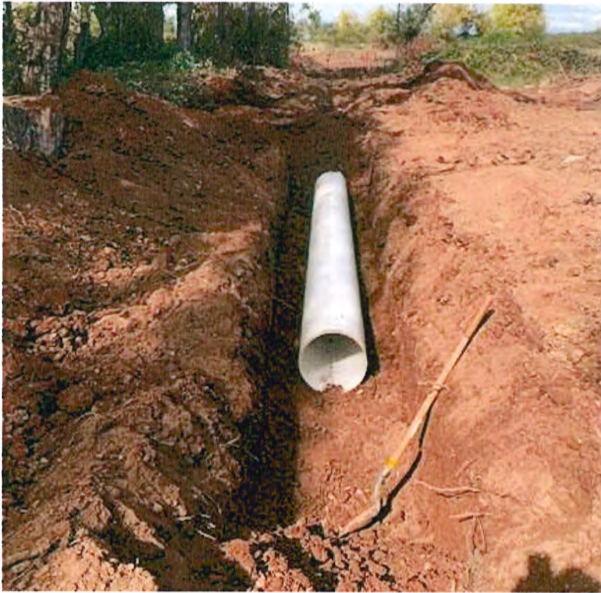
ACID replacing failed concrete pipe and open ditch
