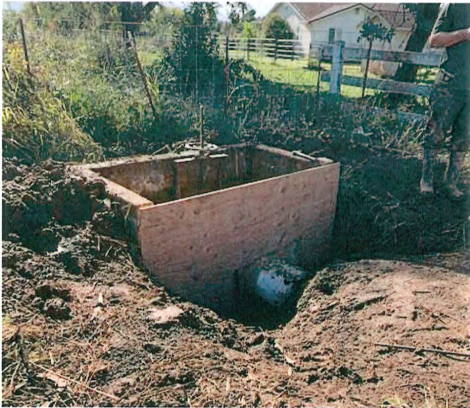
Modifying Distribution Box at Venzke Road
