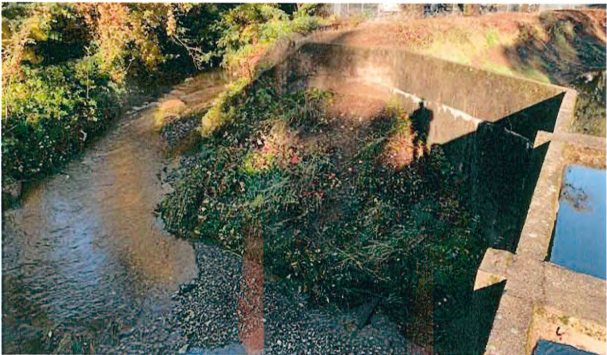
Main Canal at Oregon Gulch Vegetation Removal
