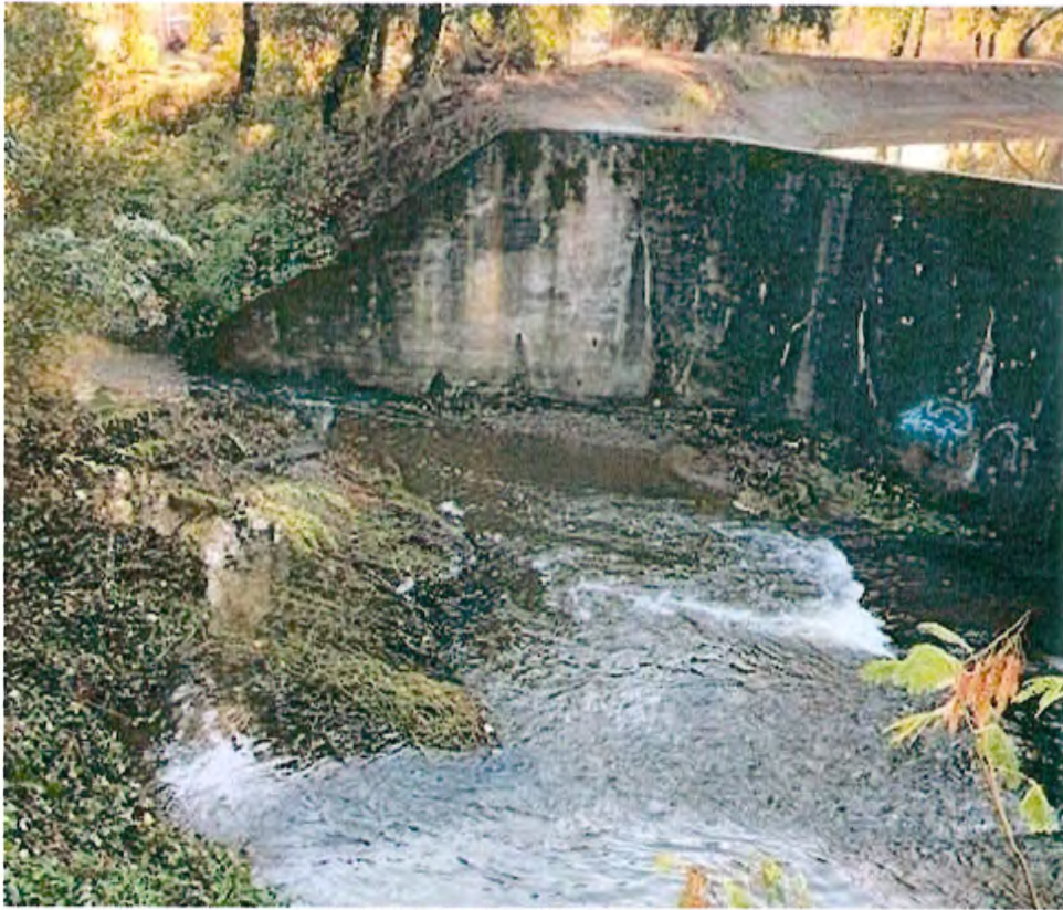
Main Canal at Oregon Gulch Vegetation Removal
