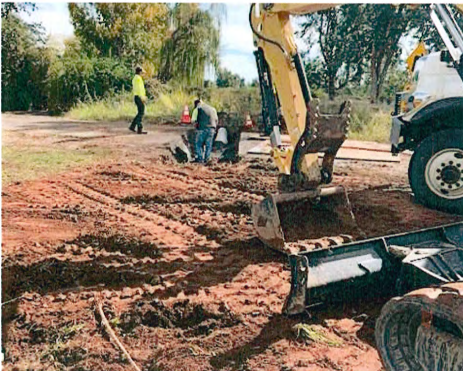
County Staff installing pipe on Venzke Road
